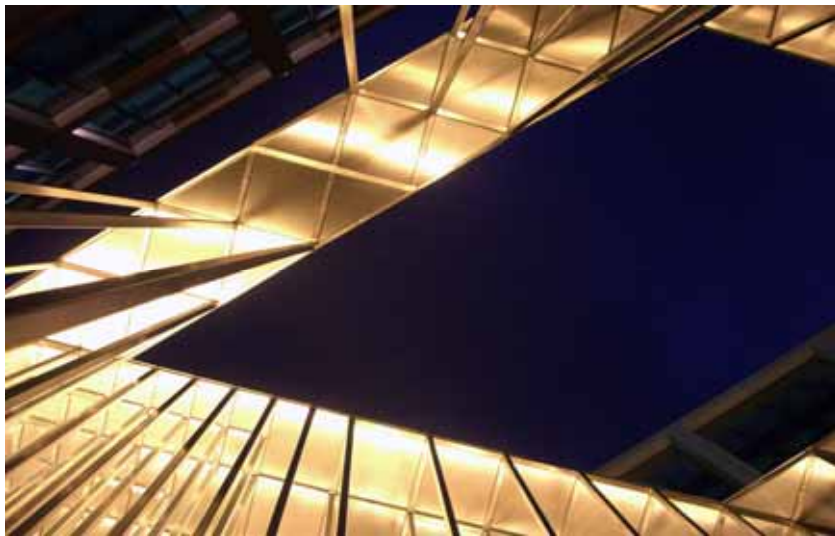
Figure 7: View of illuminated underside of roof
