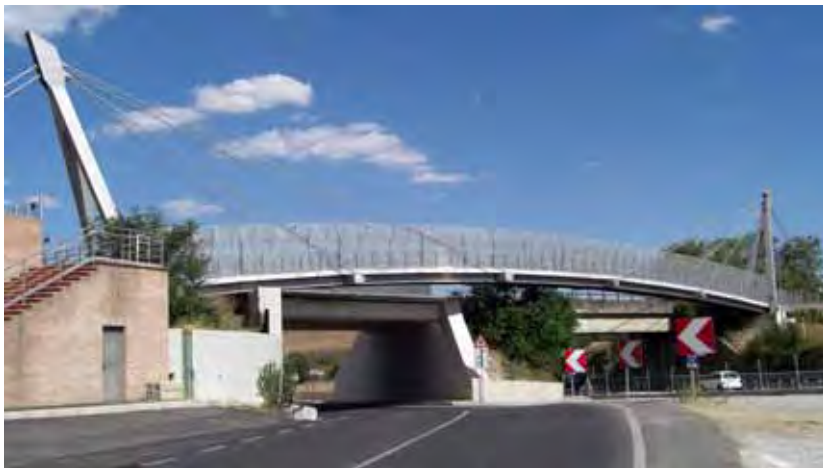
Figure 3: Highway view of the completed bridge
