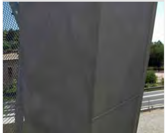
Figure 4: Welded joint on pylon
