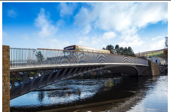
Fig 3 Replacement Pooley Bridge, using duplex stainless steel S32101 for the main structure and handrails (Photo: Outokumpu)
