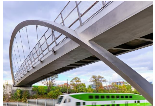
Fig 1 Garrison Crossing Pedestrian and Cycle Bridges, Toronto, Canada (Photo: Pedelta)
