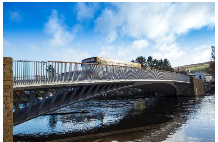
Fig 3 Replacement Pooley Bridge (Photo: Outokumpu)
