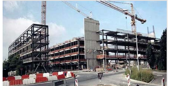
Figure 9: Erection of the structural steel framework
