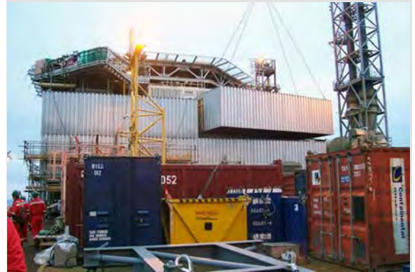
Figure 9: Installation of an accommodation module
