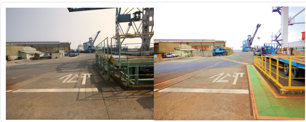
Picture 2: The safety passage – Before and after at the shipping quay
