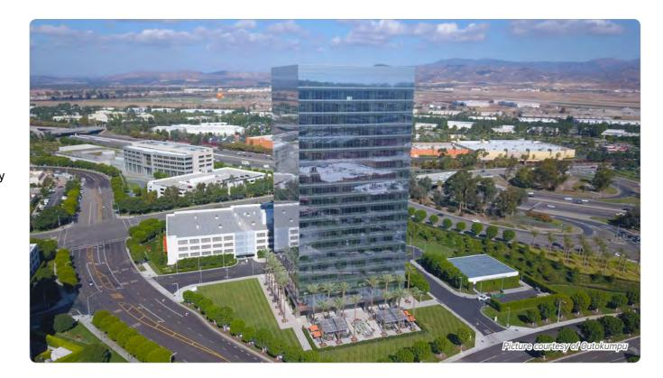
Located in the heart of Irvine Spectrum®, the building's façade is comprised of a linen-finish stainless steel and its floor-to-ceiling glass maximizes daylight and energy efficiency. Hathaway Dinwiddie also completed extensive sitework for the project.
