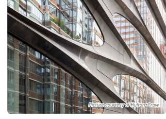
Type 304 (UNS 30400) stainless steel features a blackened finish achieved by an antiquing process, light orbital brushing and hand tinting. The panels were engineered, cut, welded and installed by Philadelphia-based fabrication group, M. Cohen and Sons. Over 350,000 man hours were invested to produce these and bring the architect's vision to life.
