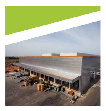
Stainless steel was selected for the roof and facade of ArcelorMittal's Sumaré Service Centre, primarily due to its aesthetic and thermal insulation properties. The fact that stainless is fully recyclable at the end of its life was also an important consideration.
