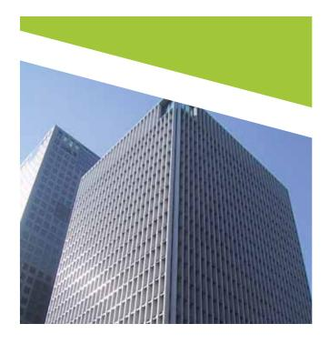
Glass-fibre-reinforced concrete (GRC) panels are light, strong and flexible, enabling them to be adapted to almost any architectural design. The GRC panels are usually attached to the building using treated metal fittings or epoxy-coated reinforced bar. For the Nippon Keidanren Building in Tokyo, ferritic stainless steel (SUS410-SD) was selected due to its high corrosion resistance, consistent quality and cost advantages.
