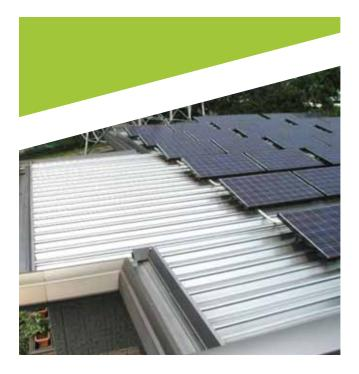
Stainless steel sheeting is being offered as an optional specification for the roofing of residential properties in Japan. This type of roofing material is in demand for use in the construction of up-market residences. The stainless steel sheeting is highly desirable due to its low carbon content. In recent years many residents have installed solar panels on their roofs. Therefore, they require roofing materials that are at least as durable as the panels themselves.
