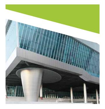
Grade STS 445 has been used in the construction of the roof and walls of the new KAIST Sport Complex building in Daejun, Korea. The use of stainless steel gives the building a feeling of grandeur.
