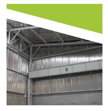
Stainless steel was selected for the roof and facade of a stainless supplier in Brazil. Stainless was chosen for its durability, thermal insulation properties, and because it is an environmentally friendly and fully recyclable material.
