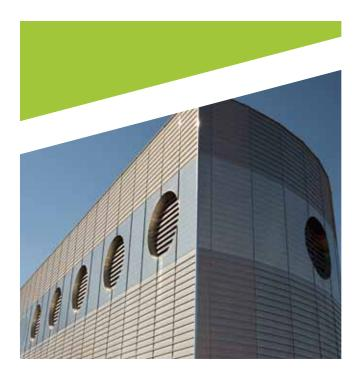
Stainless steel was chosen for this project due to its versatility, durability and sustainability. The system is composed of panels fixed on to an adjusted frame. The frame is designed to be mounted horizontally with invisible fastenings. Stainless helps to highlight the contemporary architecture of the building.
