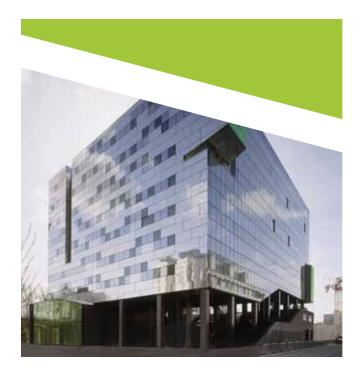
Stainless steel has been used for the gateway and streetside facade of this office building in Paris. The use of stainless with a bright annealed finish creates a play of light on the façade. The combination stainless steel and clear and coloured double-glazing, echoes the reflections of the nearby Seine River.
