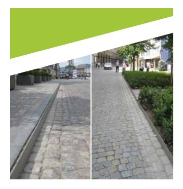
Stainless steel borders provide an unusual yet attractive feature to separate pavements from planted areas in the historic city of Mechelen, Belgium. Not only do the borders save space, but they are also virtually maintenance free. Permanent contact with soil and concrete foundations, and occasional exposure to de-icing salts, were some of the factors taken into account when choosing the grade of steel to be used for the border.
