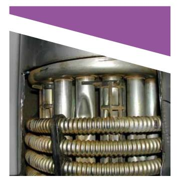
The use of stainless grade SUS304 with copper (Cu) and tungsten (W) inhibits pitting in these boiler tubes. Pitting causes localised small holes in the metal which weakens the structure.
