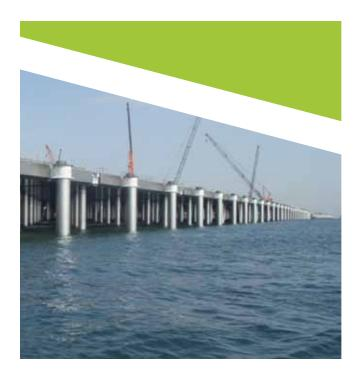
The expansion of Haneda Airport in Japan has required the construction of a new runway over the sea. Stainless steel has been used to protect the pillars that support the runway. The decision to use stainless steel was based on its durability and high-resistance to seawater corrosion. Both of these factors give stainless steel a superb lifecycle cost advantage.
