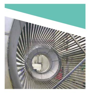
Welded or seamless stainless steel tubes are used for this heat recovery exchange system in a hot rolling steel mill. Seamless tubes are used for recovery systems that are fed by hot air (above 450°C). If the system is fed by cold air (up to 450°C) welded stainless tubes suit the requirements of the plant's maintenance department.
