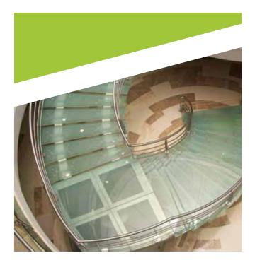
The construction of this staircase in the stylish new Moksha Plaza shopping mall in Mumbai utilised 4.5 tonnes of stainless steel grades SS304 and SS316. Several forms were utilised including spiders, trapezoids and tubes.
