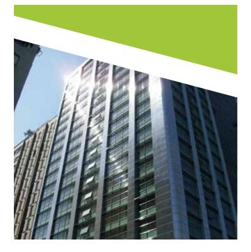
This office building is located 2 km from the sea and required extensive renovation. The existing masonry facade was replaced with a new curtain wall consisting of stainless steel cladding and solar shade elements. The frame of the external cover was made with AISI 444 grade stainless which can withstand the corrosive effect of the nearby sea.
