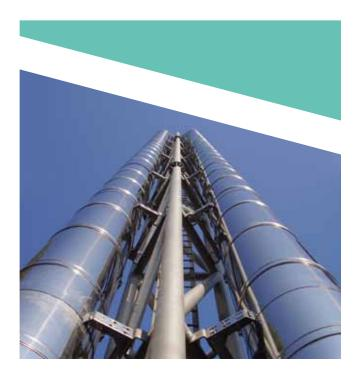
External chimney flues have traditionally been made with stainless steel grades such as AISI 304 or 316. However, ferritic stainless grades such as AISI 441 or 444 offer significant advantages. These include price stability over the longer term due to the low-levels of expensive alloys found in non-ferritic grades.
