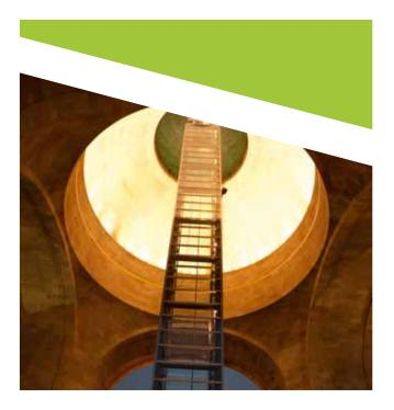
Renovations to Mexico City's *Monumento a la Revolución* were undertaken to commemorate the 100<sup>th</sup> anniversary of the Mexican revolution. Part of the work involved the construction of this stunning new elevator structure inside the monument. Built with a stainless steel frame, the elevator stands at 50.7 metres high. Stainless steel was also used in the construction of hand rails for an adjoining staircase, and in the museum located in the basement of the monument.
