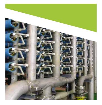
In brackish-water desalination plants (BWDP) the use of AISI-316L SS in the feed side and AISI-904L in the brine side of the reverse osmosis train is required to avoid corrosion and to provide mechanical resistance to the fluid operating pressures.
