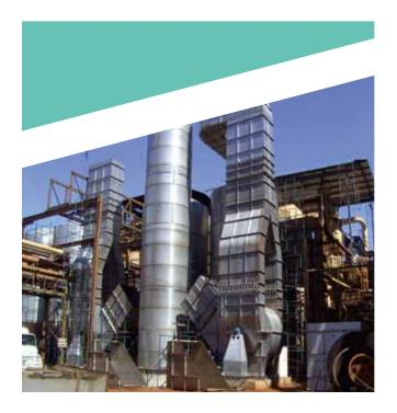
Gas washers are used to clean particulates and harmful chemicals from the exhaust systems of factories. Once the exhaust is washed, the clean air can be released into the atmosphere.
