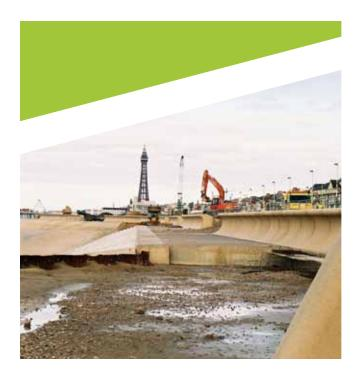
A three kilometre sea defence wall was constructed to protect the city of Blackpool in the north west of England. Stainless steel reinforcing bar was used instead of carbon steel reinforcing bar in critical areas. This allowed concrete coverage to be reduced in these places, but will still guarantee a long service life for the protective wall.
