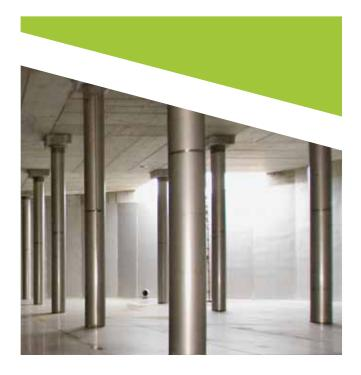
Two large tanks (6 m high, 31 m diameter) were installed to store drinking water for the town of L'Aquila in Italy. Thanks to the Aquawall technology adopted for this project, the tanks could be completed and installed in only 18 days. Three days were required to erect the prefabricated walls, while the remaining 15 days were devoted to the vertical welding of the walls and the installation and welding of the tank bottoms.
