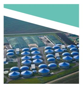
An agricultural biomass energy generation plant generates thermal energy for use on the farm. Excess power that is not required can be fed into the national electricity grid. The heart of the system is the fermenter where the biomass is broken down. The liquid and gases inside a fermenter are very aggressive. As a result, the tanks must be constructed from corrosion-resistant materials such as stainless steel.
