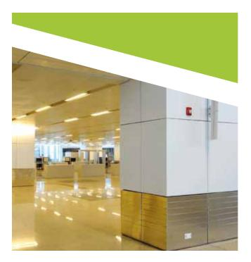
With an area of half a million square metres (5.4 million feet<sup>2</sup>), Delhi's new airport terminal is one of the largest in the world and is expected to handle 34 million passengers annually. The pillars of the terminal are clad in 5,000 m<sup>2</sup> of stainless steel - just one of many examples of the use of stainless steel inside the new building. Stainless steel was selected because it provides a classic finish while remaining hard-wearing and easy to maintain.
