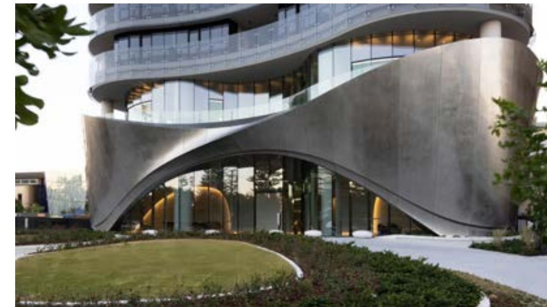
272 Hedges Avenue Pedestal Residential Building. Pictures © Peter Sexty
