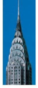
Although it has only been cleaned once, the stainless steel roof of the Chrysler Building is still in excellent condition after more than 70 years.
