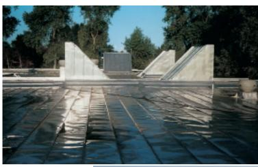
A standard 2B mill finish offers a particularly costeffective solution for flat roofs.
