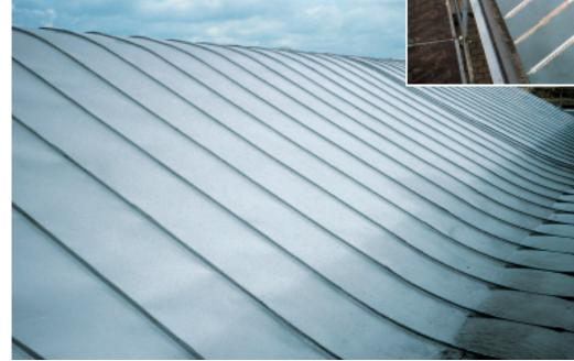
Welded roofs can be used on most roof geometries.
