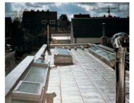
Welded stainless steel is typically used on flat roofs with little or no slope for which no other metallic solution is appropriate.
