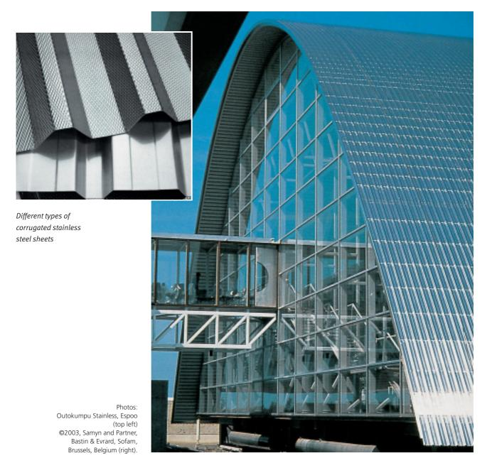
Stainless steel profiled sheets with greater section depths are used for structural roof decking. These support different kinds of flat or pitched roofs where the environment within the building is corrosive e.g. paper mills, water purification plants, breweries or composting plants.
