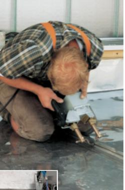
Portable spot welding equipment
