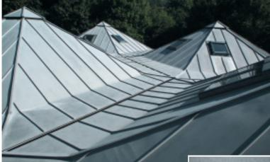
Electrolytic coating on both sides with a very thin layer of 100% tin. The advantage of this tin layer is not only the matt grey appearance, but it simplifies the soldering of finishing pieces, such as gutters, roof penetrations and flashings. Accessories are readily available in this finish material.
