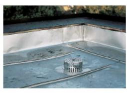
Custom-made gully (top), installed gully complete with strainer (bottom).
