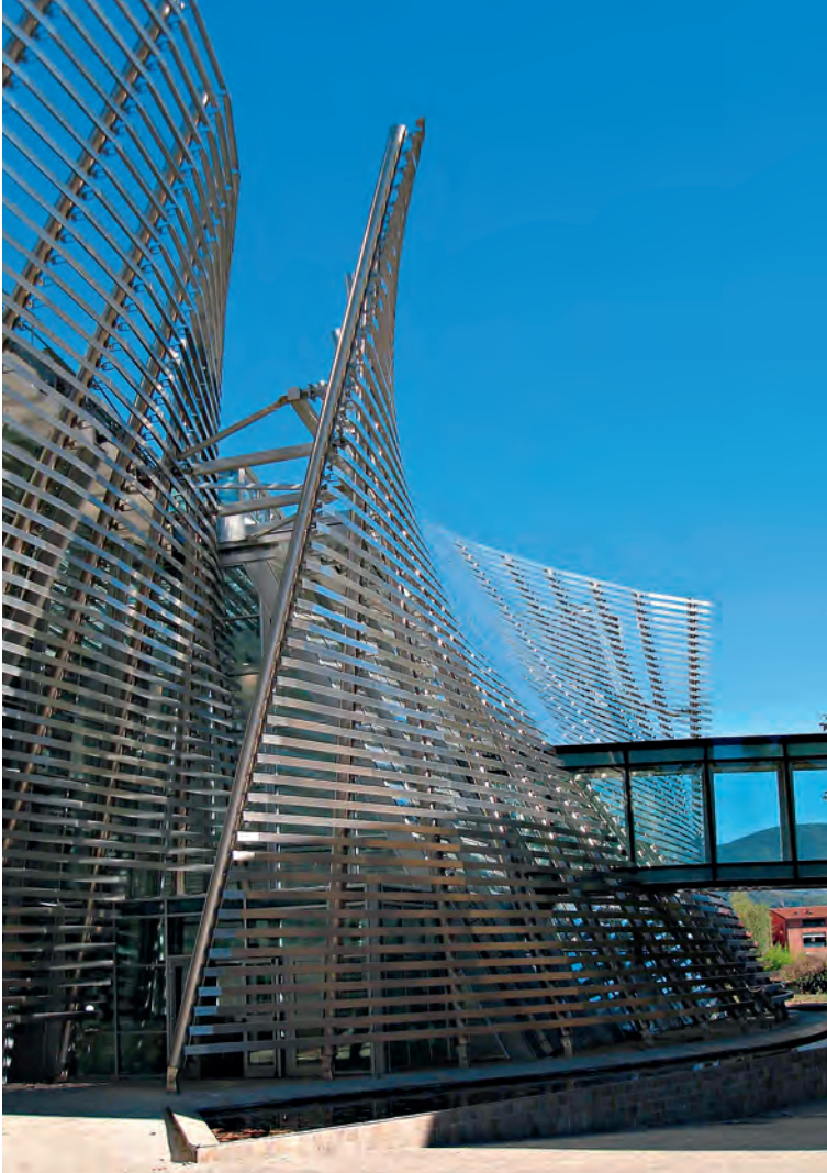
The entrance to the law courts lies between the two overlapping parts of the external solar shading.
