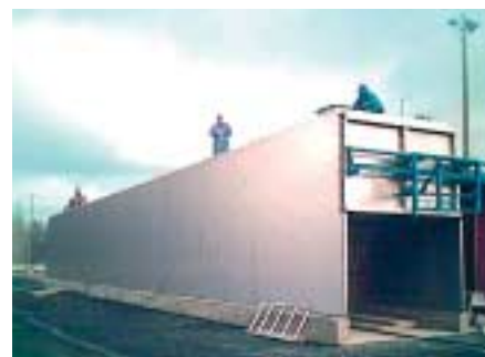
Figure 6. Stainless steel sandwich panels made of austenitic stainless steel grade 1.4301 (AISI 304) used in the wood drying tunnel. (Photo: Kennotech Oy)
