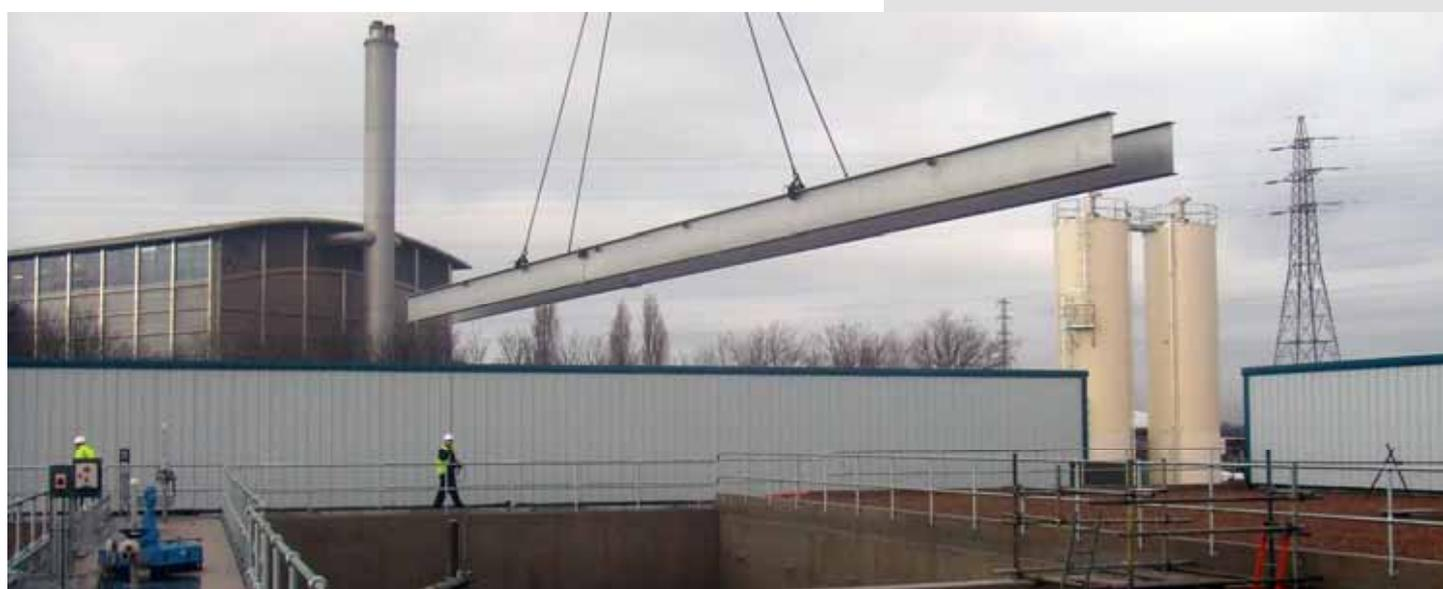
Figure 8: Installation of a pair of main beams
