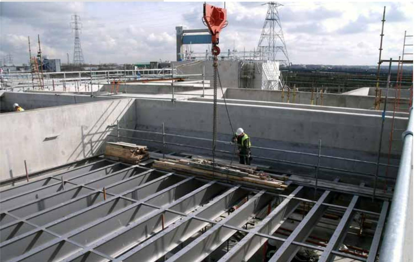
Figure 7: Completed lamella steelwork
