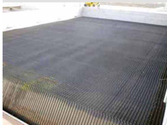
Figure 4: Lamella clarification filter
