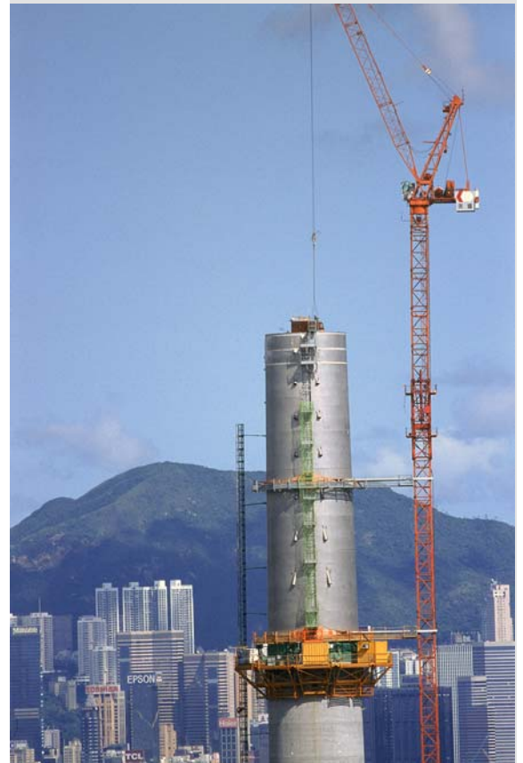
Figure 7: Installation of stainless steel skin segments
