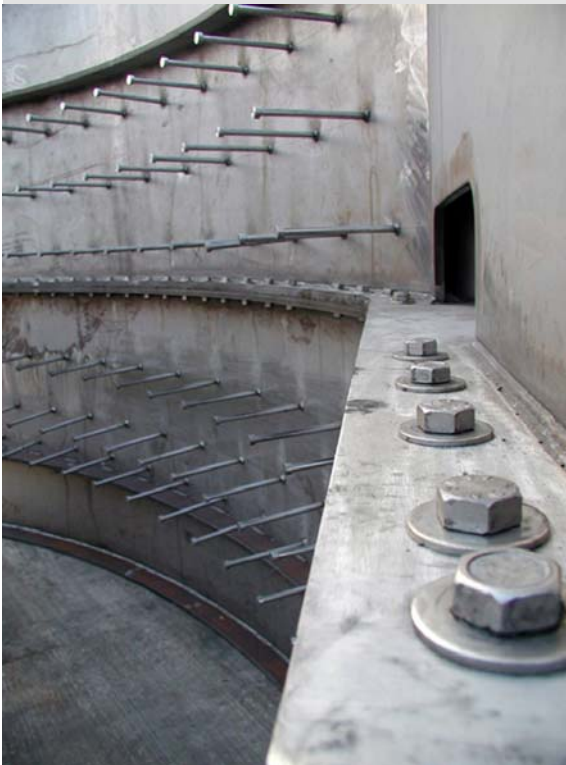
Figure 6: Edge flange connection
