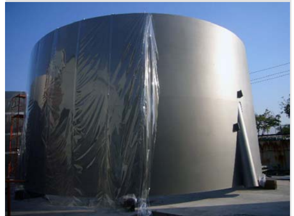
Figure 3: Segment of stainless steel skin
