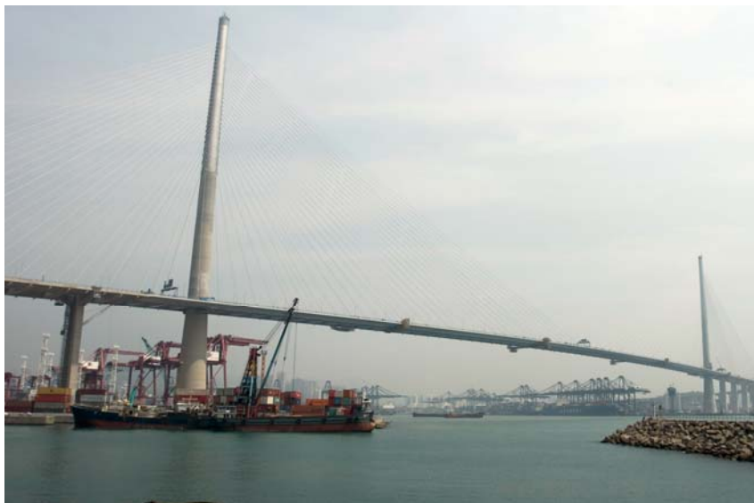
Figure 1: General view of Stonecutters Bridge
