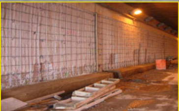
Kevin Cornell/Salit Specialty Rebar
