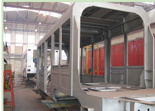
Fabrication of Tango light rail carriages in the workshop (Photo: ThyssenKrupp Nirosta)
