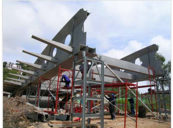
Figure 11: Temporary supports for the main structure
