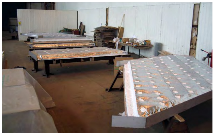
Figure 7: Insulation placed inside the wall panels
