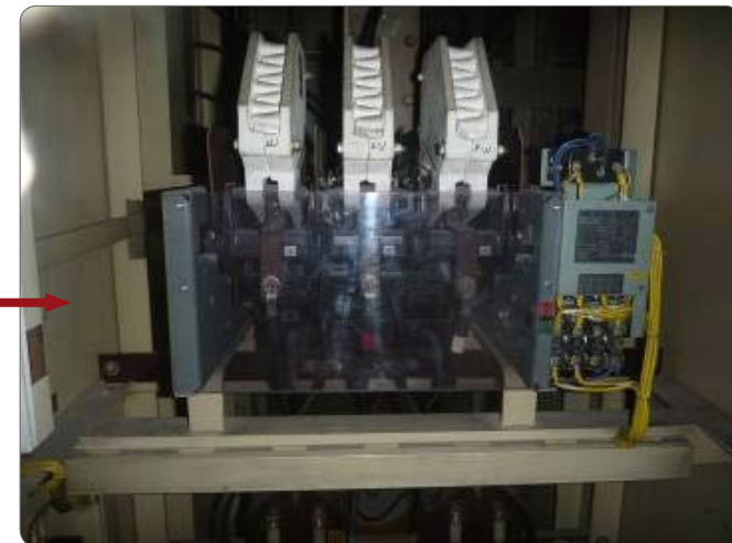
Installing the insulation to the bus bars
