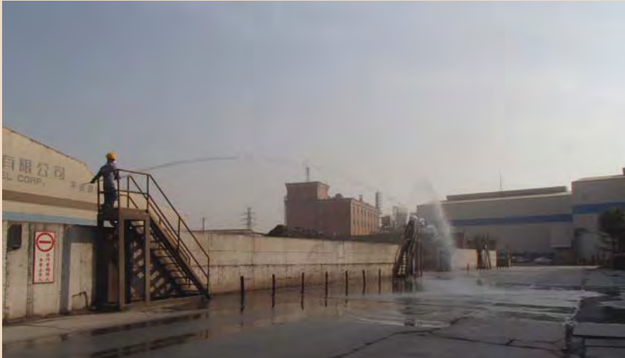
A series of 33 overlapping fire hydrants have been installed along the vehicle's path in case of a slag splash during transportation
