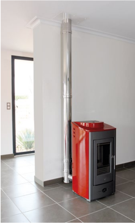
Stainless steel chimneys contribute to the clean burning of modern fuels – including pellets, which are growing in importance as renewable sources of energy. Photo: Poujoulat, Saint-Symphorien (F)
