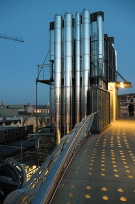
Chimneys are subject to harmonized European standards.
