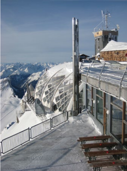
Stainless steel chimneys are a symbol of efficient and clean heating.
