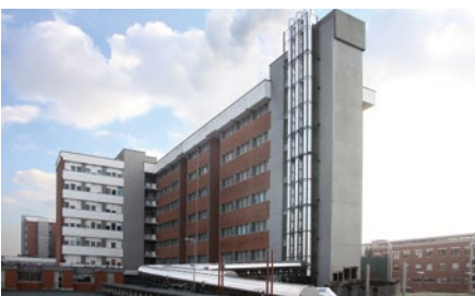
Double-walled, thermally insulated external chimneys were originally conceived for renovation. Photo: Roccheggiani, Camerano, Ancona (I)
