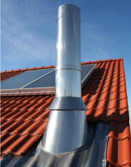
Chimney manufacturers provide insulation sleeves for roof penetrations, which eliminate fire risks. Photo: Schiedel, Vienna (A)
