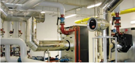
Stainless steel flues are resistant to the acidic conditions created by condensing boilers. Photo: Poujoulat, Saint Symphorien (F)
