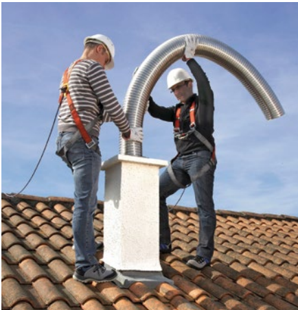
Flexible liners are a preferred refurbishment solution because they are quick and cost-effective to install. Photo: Poujoulat, Saint-Symphorien (F)
