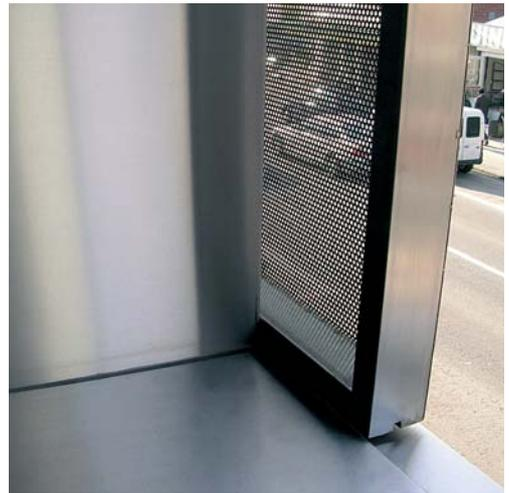
*The perforated stainless steel of the sliding panel retains a visual connection with the outside while also protecting against direct sun.*
