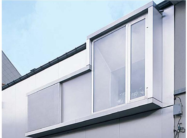
*The projecting window assembly adds relief and depth to the façade.*
