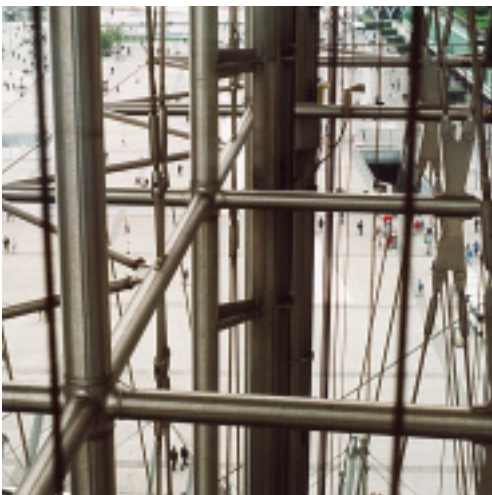
The design of this particularly lightweight and transparent lift bank was based on the high performance provided by stainless steel.
