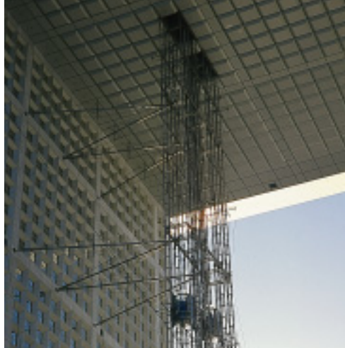
The minimalist web-like metal lift cage structure ensures a panoramic view from the cars.
