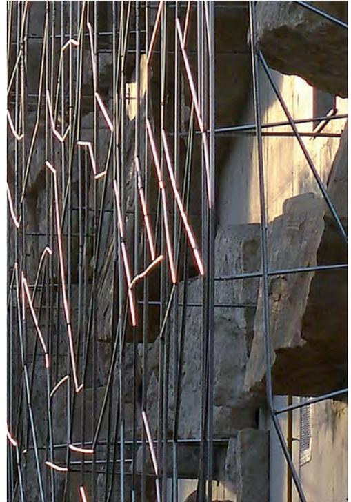
*A grid of 20 mm welded stainless steel tube overlays the concrete walls inset with stone blocks.*
