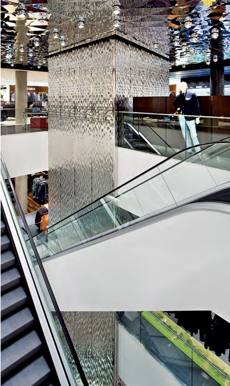
Light bounces off the mirror-polished stainless steel cladding on the lift core, creating a waterfall effect.
