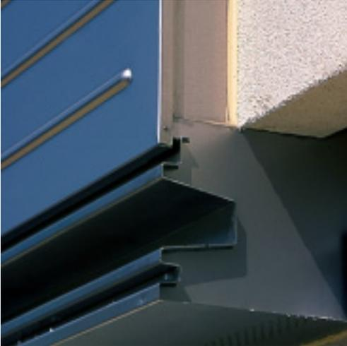
“The panels are stamped from a form, implying set dimensions. But given that, by definition, a building grid is never completely standard, we had to appreciably vary the panel lengths when laying the cladding, although the tops remained fixed.
