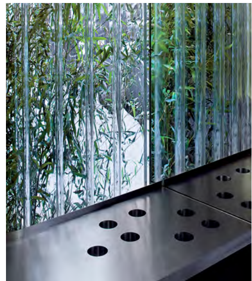
Bamboo plants growing up from the basement are visible in the glazed street front and in the ground-floor customer area. Stainless steel sheet, bent to shape, was used for the bench wrapped around the curve of the glass partition.
