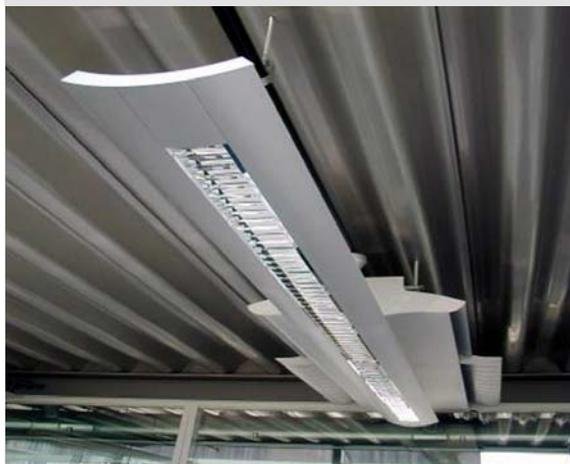
Figure 6: Lighting and air distribution units suspended from the profiled decking
