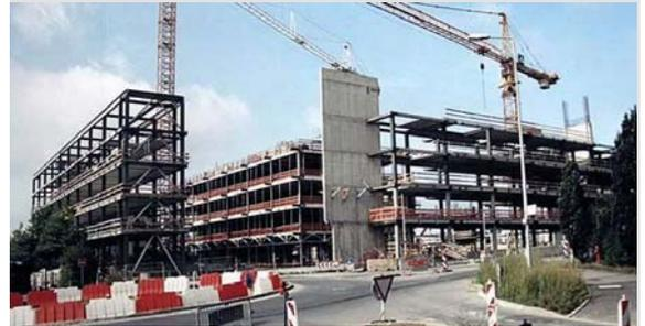
Figure 9: Erection of the structural steel framework
