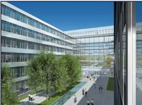
Stainless steel panels (Grade 1.4404) are attached to the outer walls of this 6-storey office building in Hannover (Germany) using an adhesive bonding system without the need for additional mechanical fastening
