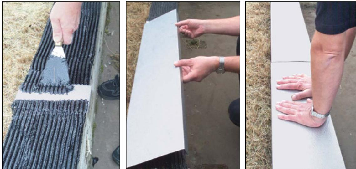
Adhesive bonding is a practical solution in building applications, when stainless steel has to be fastened to masonry or natural stone
