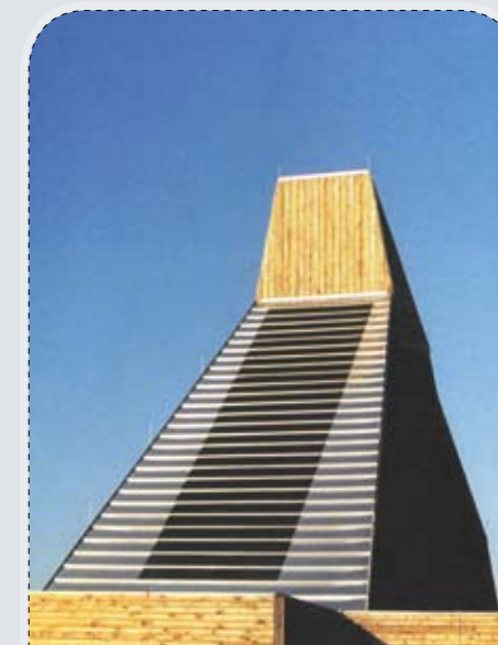
FIGURE 1: The tilted stainless steel roof of the German Nautical Museum in Stralsund with integrated photovoltaic modules
