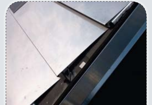
FIGURE 6: Multifunctional photovoltaic roofing elements at the assembly stage
