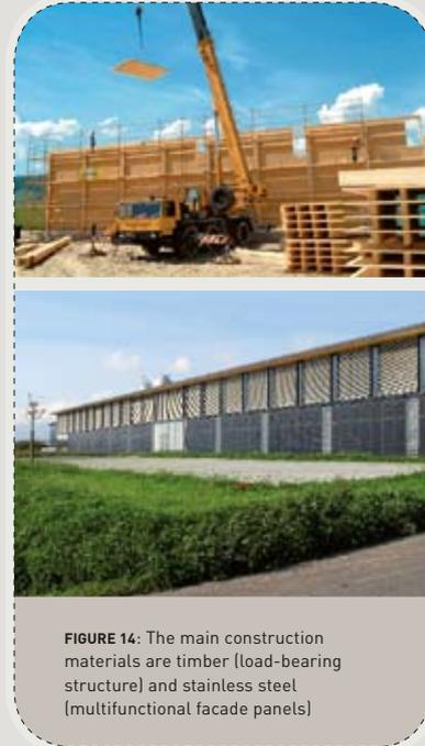
**FIGURE 14:** The main construction materials are timber (load-bearing structure) and stainless steel (multifunctional facade panels)
