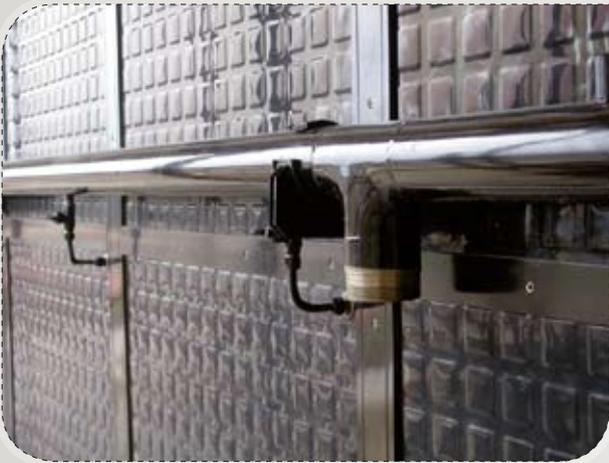
**FIGURE 12:** Close-up of the connection of the collectors to the upper tube for heat transfer fluid
