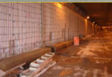
Kevin Cornell/Salit Specialty Rebar
