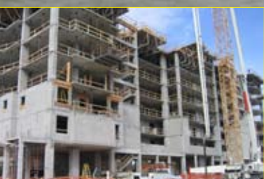
Kevin Cornell/Salit Specialty Rebar
